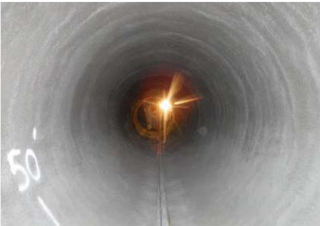
Rehabilitated pipe after EcoCast installation
