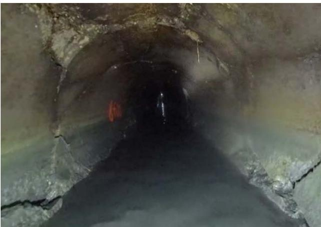
Manned walkthrough inspection of the deteriorated interceptor
