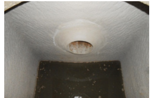
Manhole renewed using the EcoCast geopolymer lining system.
