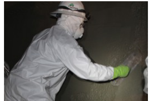
Trowels are used to smooth the finish flat surfaces.
