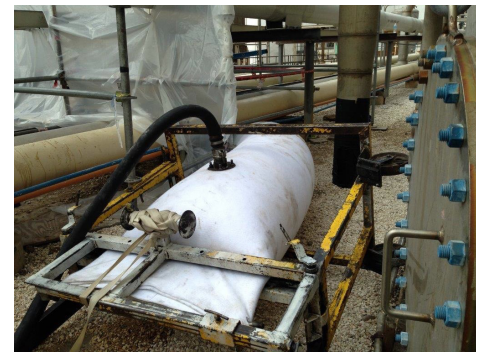
CIPP liner above ground at inversion point.
