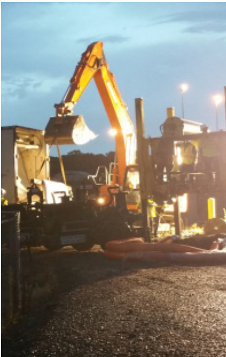
CIPP Preparation site
