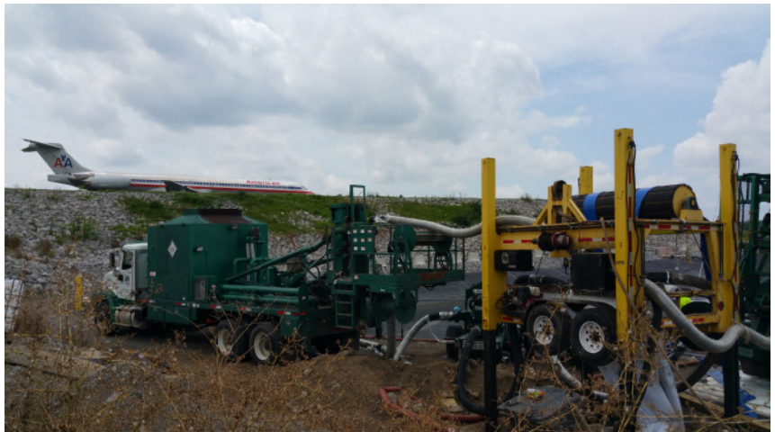
CIPP is being prepared for curing process
