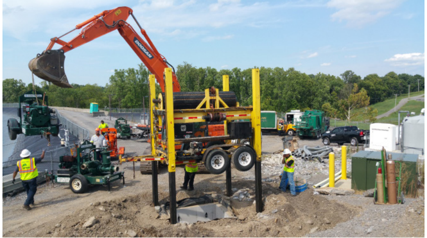
Preparation of the CIPP inversion process
