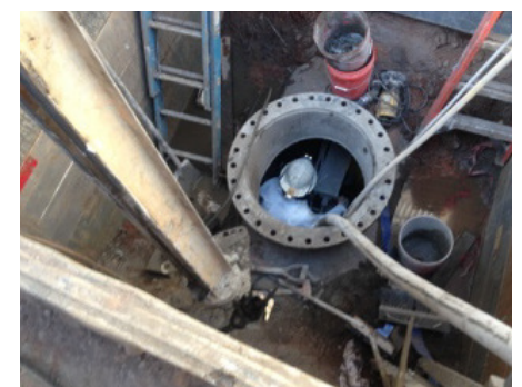
A 30" man-way was cut into the cooling line to gain access.
