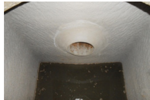
Manhole renewed using the EcoCast geopolymer lining system.
