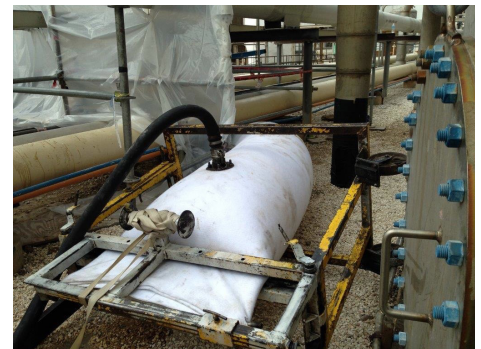
CIPP liner above ground at inversion point.
